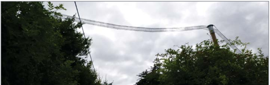
Above: Picket Piece dormouse bridge over Ox Drove
